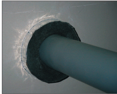
Fire stopping of insulated pipe penetrations
